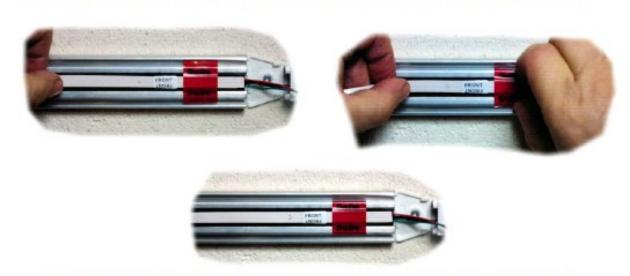
Repeat the procedure fixing mounting stickers about every 150mm to 300mm. Ensure the mounting stickers do not obstruct the LEDS
